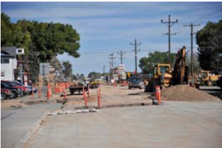
Douglas fuel tax project under construction.
